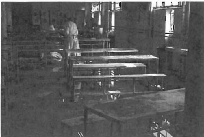
Flooded kitchen caused by defective water tanker
