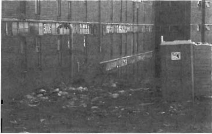
Rubbish and raw sewerage (from portable toilets installed for informal settlement) accumulating against outside wall of hostel
