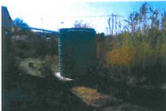
“PHOTO 3” (ANOTHER WATER TANK)
