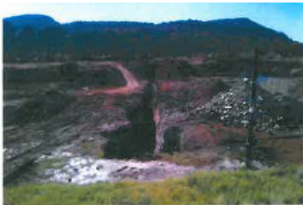
“PHOTO 4” (Construction at Jagersfontein of water pipes from Kalkfontein Dam)
