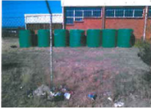
“PHOTO 1” (PHOTO REFLECTING EMPTY WATER TANKS WHICH HAVE NOT BEEN FILLED WITH WATER)
